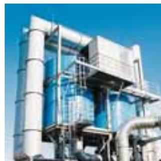
Hot, dust-laden oxy-fuel gases, produced, for example, when breaking up slag-blocks or cast blocks from converter or blast furnace smelts, are effectively captured, exhausted and dedusted before they are discharged into the atmosphere.
