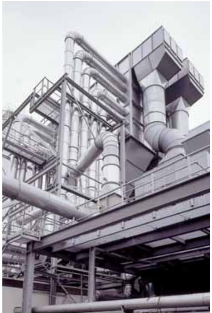
When ducts carrying material pass through fire protection barriers, safety elements, such as quick-closing fire-gates or fire protection dampers, can be used to isolate individual fire sections from one another.
