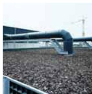
The supply scope also includes the treatment of odorous air or air containing carbon. As well as classical bio-filters, bio-scrubbers with trickling filters can also be used.
